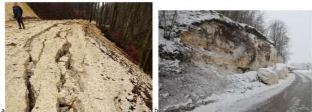
Figure 7. Coseismic landslide activation: a) slide in forest road embankment (near Strašnik, observation point ŠP-3); b) rockfall near Pečki that blocked the local road (observation point IK-ODR).
